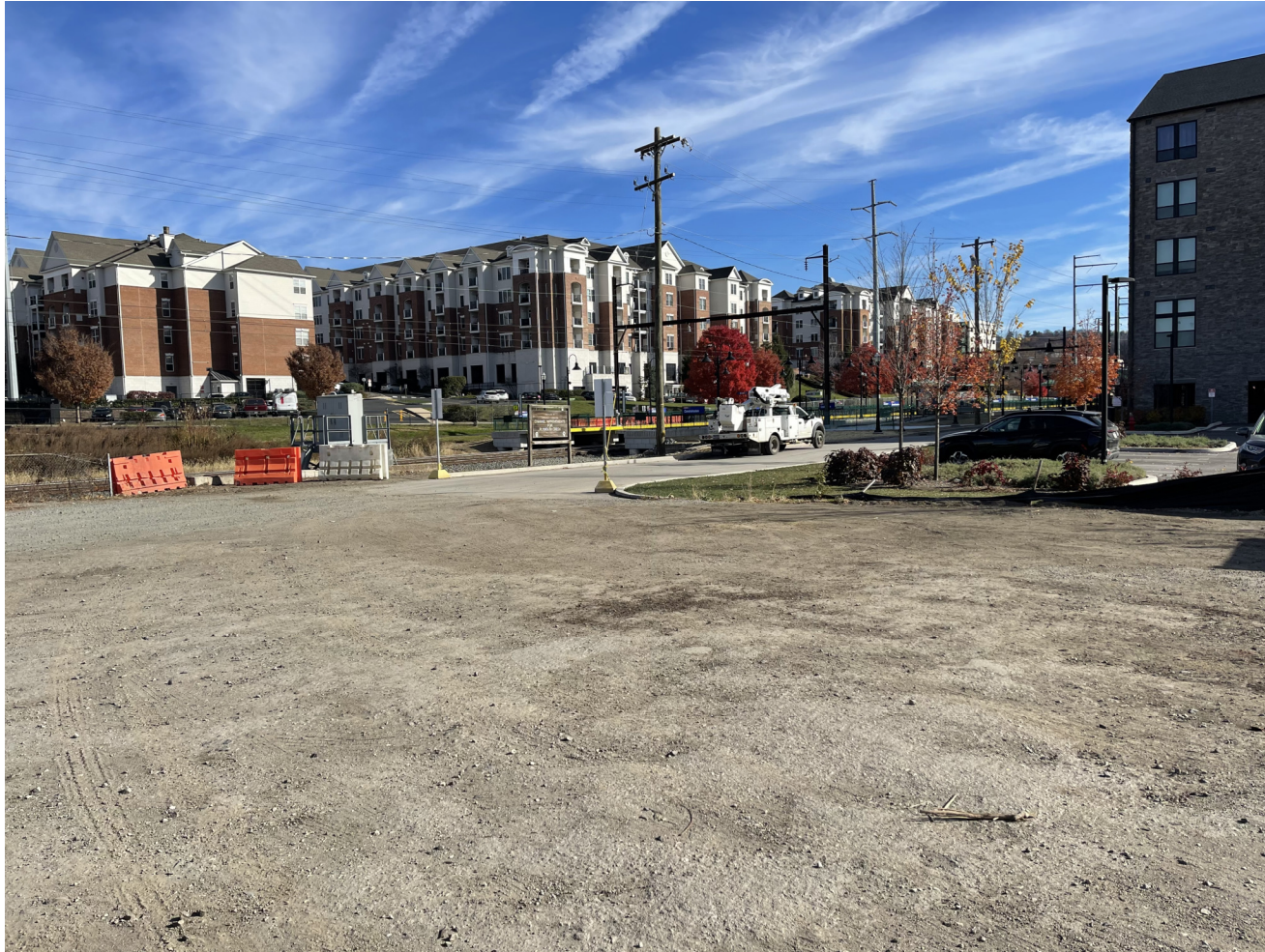
Photo 1 – Looking East towards the Access Road entrance to the site
