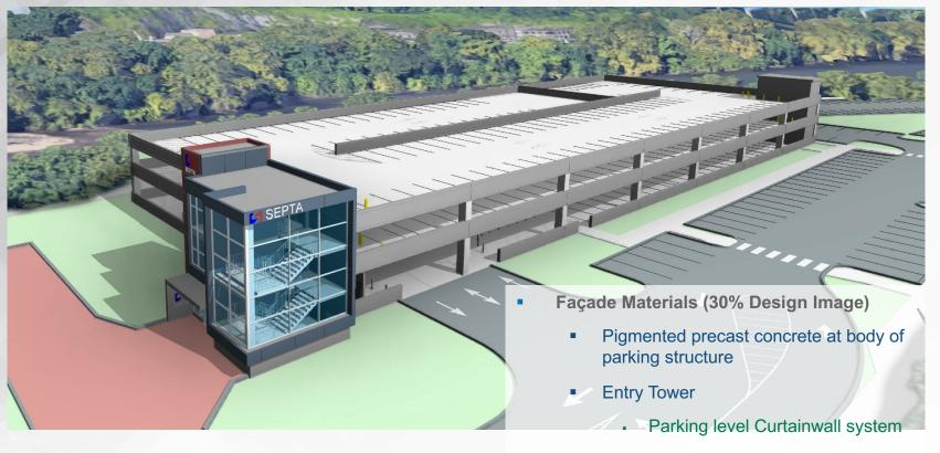
Pigmented precast concrete with thin brick cast via form liner
