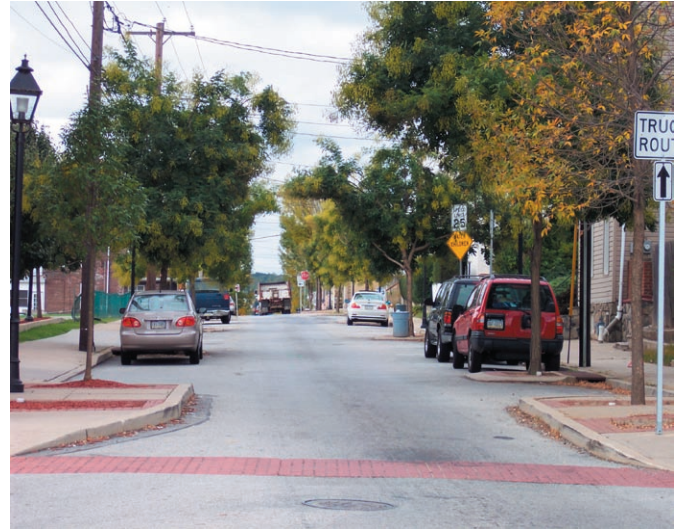
Curb-extensions on Hector Street
