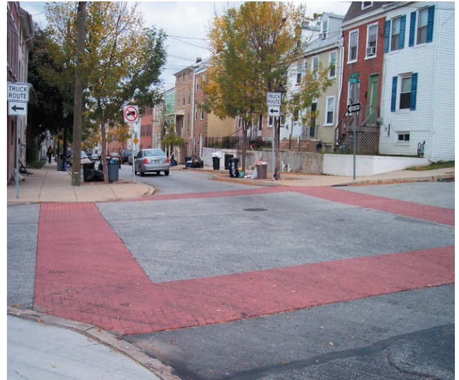
Streetscaping upgrades along Hector Street
