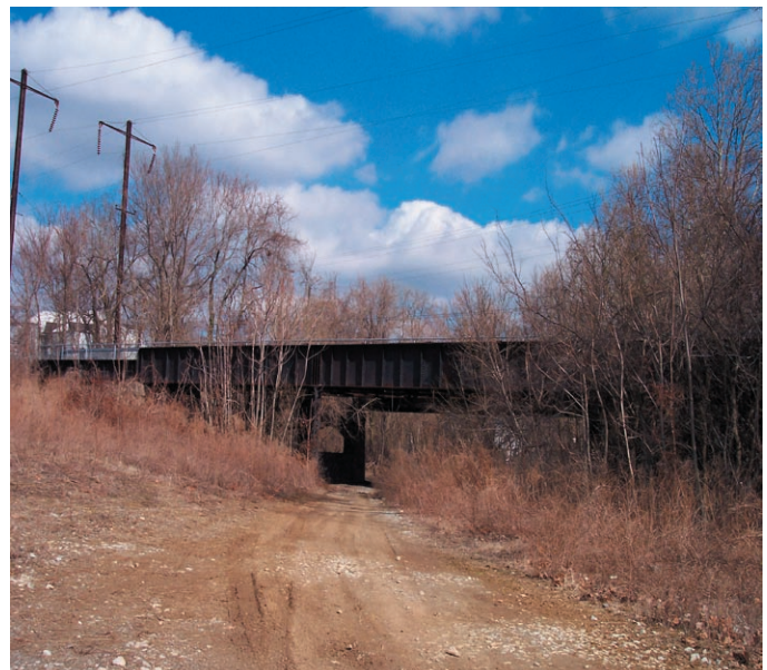
Schuylkill River Trail Bridge over future Plymouth Trail location
