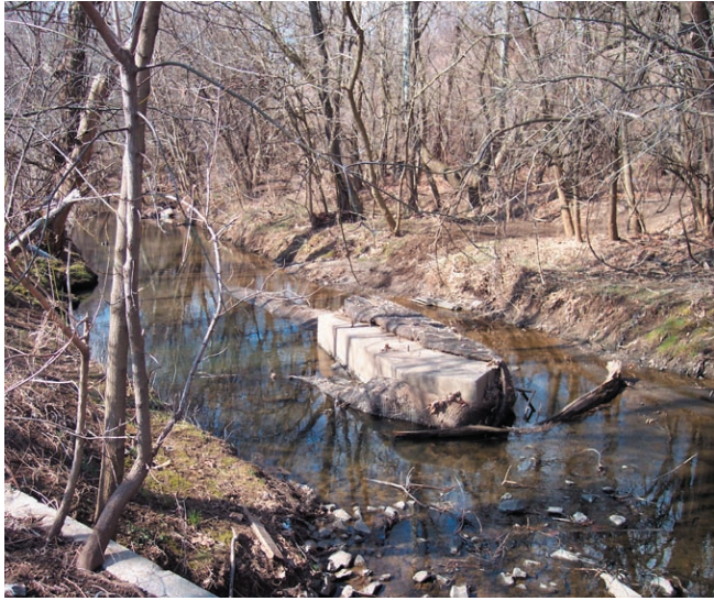
Existing bridge footing in the Plymouth Creek
