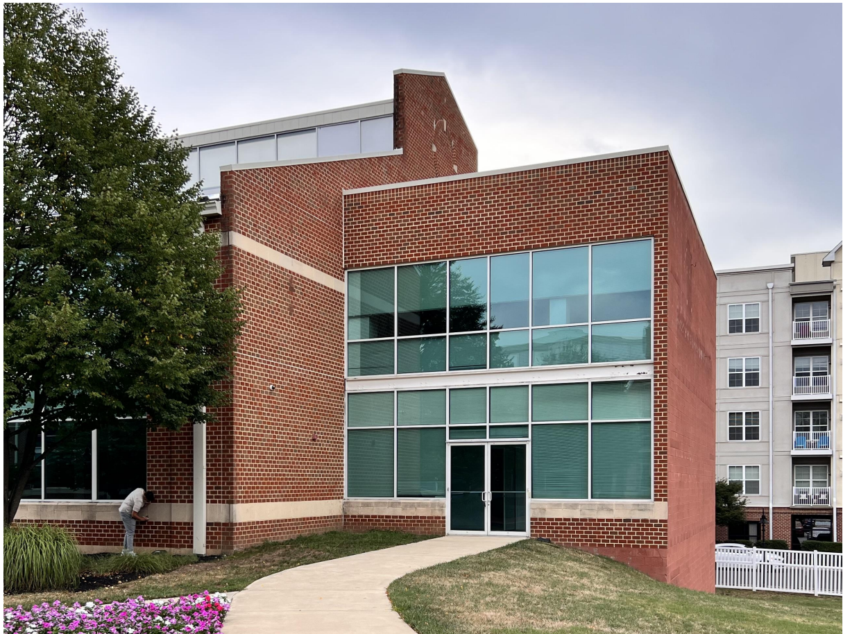
MORGAN PROPERTIES - EXISTING CONDITIONS
