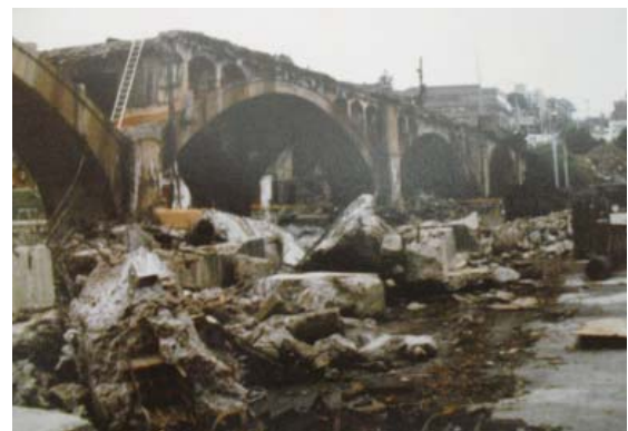
Demolition of the prior Matsonford Bridge, c. 1984
