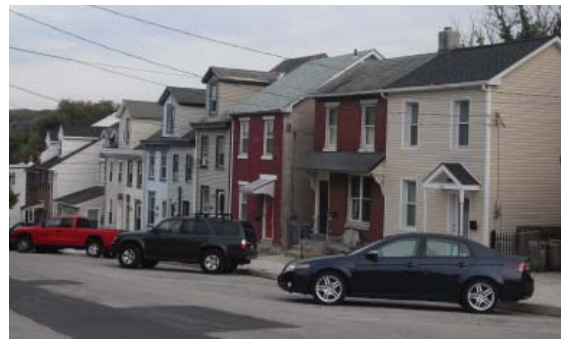
Worker housing along Spring Mill Avenue
