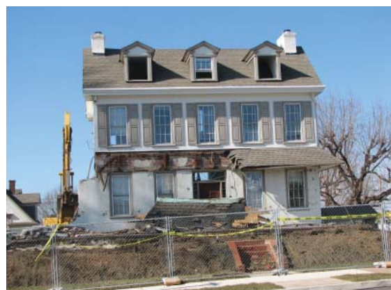
528 Fayette Street during demolition in March 2011
