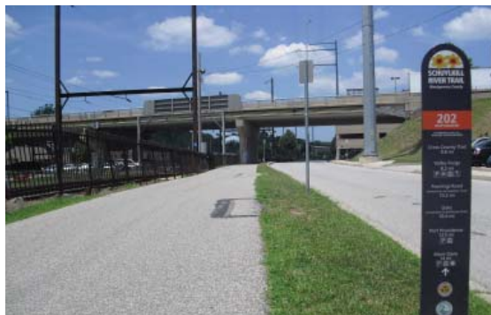
Matsonford Bridge (background) and Schuylkill River Trail (foreground)
