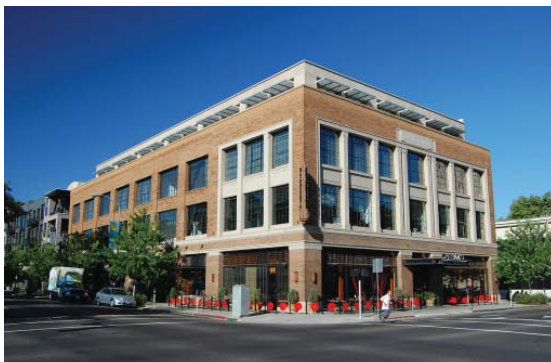
Pedestrian-oriented commercial infill in Sacramento, CA
