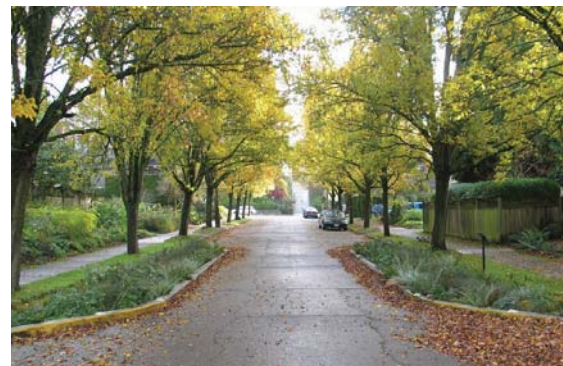
Stormwater management bump-outs in Portland, OR
