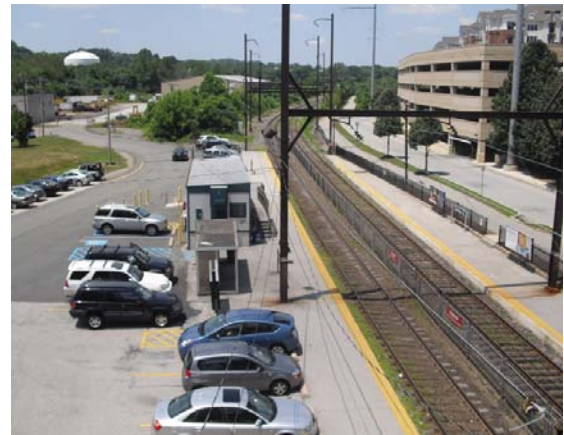
Current train station conditions
